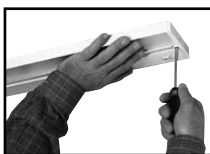
Step 3 Mount fixture to cabinet bottom using captive mounting screws.
